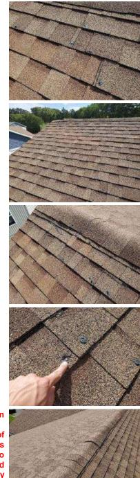
Building 9. Ridge vent appears to have been eliminated to separate the attic spaces.
