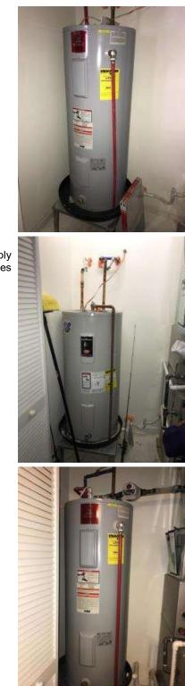
7101. Recently installed. Sediment in drip pan. Corrosion noted on the supply lines. Monitor for potential leaks on the supply lines and make repairs as needed.
