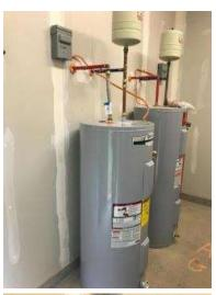
5205, 5202 Corrosion periodic leaks are occurring most likely due to a flooded expansion tank.
