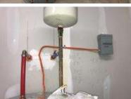
4203. Corrosion periodic leaks are occuring most likely due to a flooded expansion tank.
